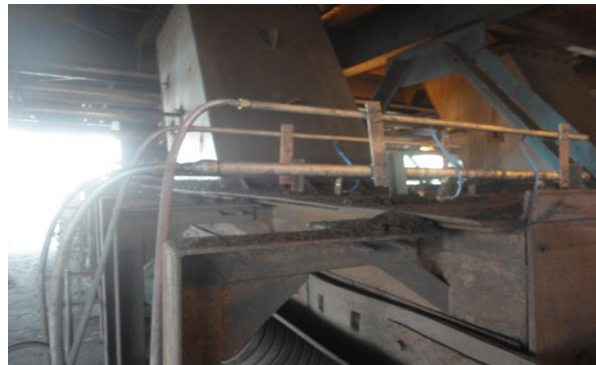
Fixed type dust suppression system
