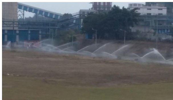
Fixed type dust suppression system
